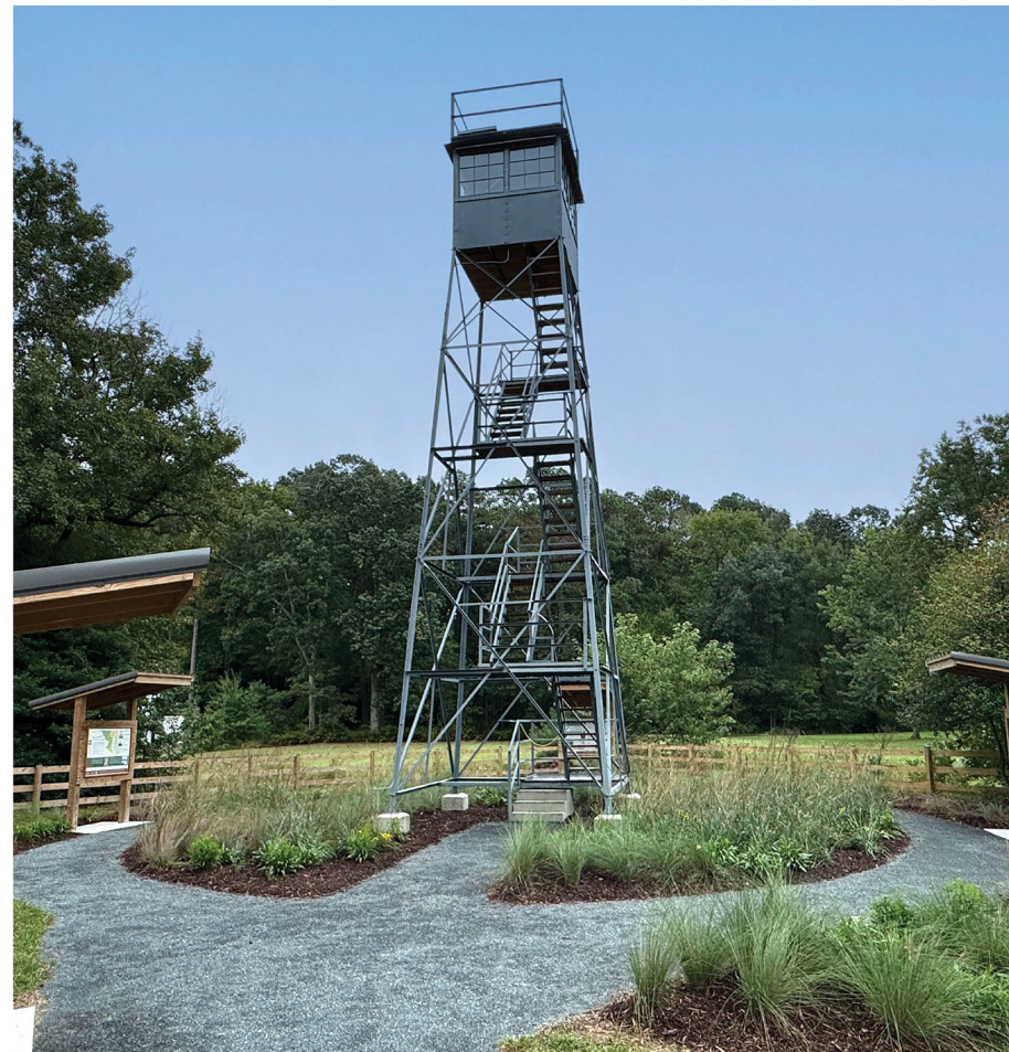
Tower and Park Overview (Looking East)
